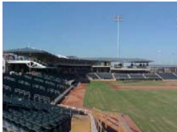
Overall view of Stadium. Club seating being installed
