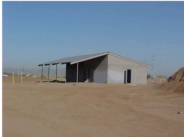
Avondale Youth Sports Complex restroom/concession building ready for painting & fixture install.
