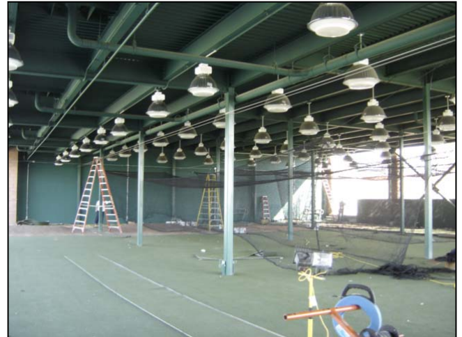
View of new batting tunnel
