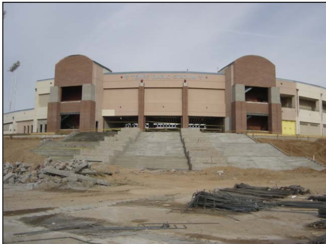
Progress on the grand stairway
