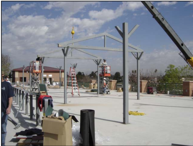
Steel erection underway for the Charro's pavilion located in right field
