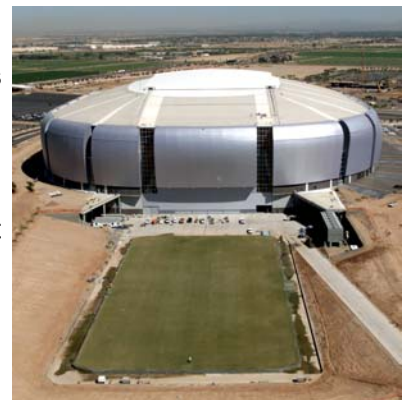
Soak up the Sun — The natural grass field sits outside 95% of the year allowing the floor to be used for tradeshows, conventions and other non-football events.
