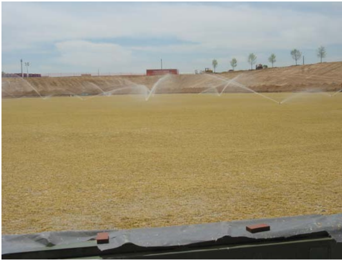
Special Turf for a Special Field — The newly installed stolons on North America's first roll-in field get watered from the field tray's internal sprinkler system. The stolons, which first appeared tan after planting, were set into a special sand-based root zone mix. The turf is called "Tifway 419" which thrives in Arizona.
