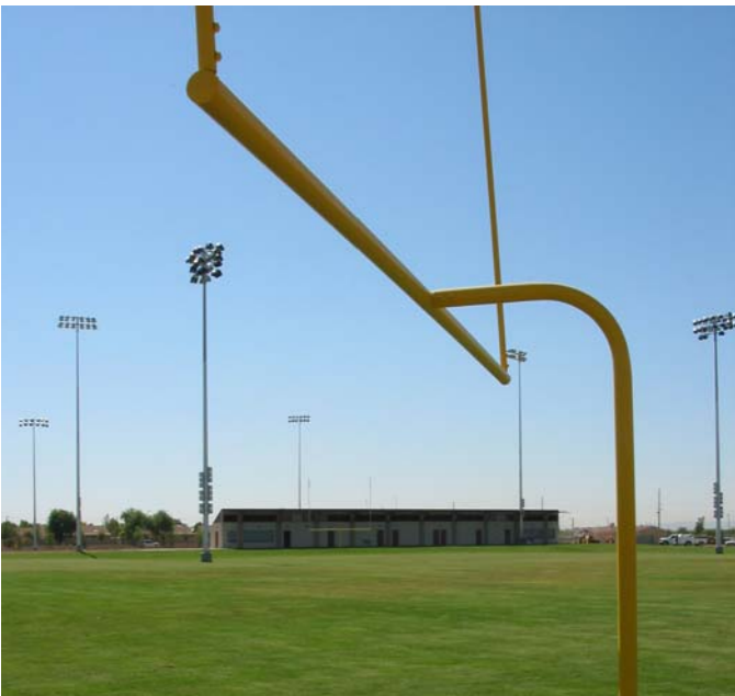
Glendale Youth Fields Near Stadium — The first phase of the project, funded with $1 million from AZSTA, contains 5 fields.
